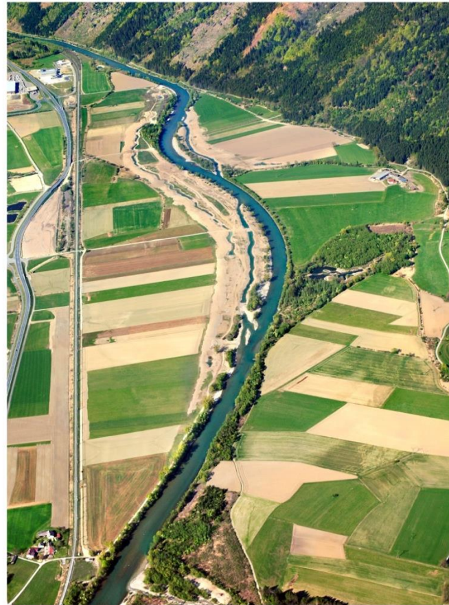
Baufortschritt Flug v. 20.April 2011
