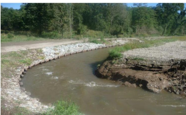
Dokležovje, Bank revetments removal; new side channel;
